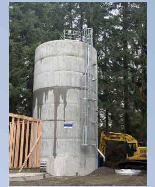
Fully constructed reservoir
