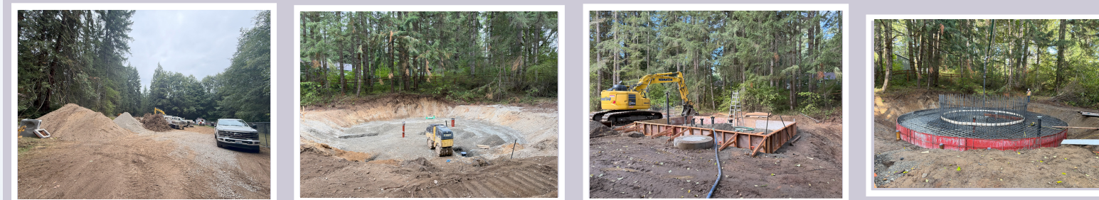
Construction site for 90,000-gallon concrete reservoir and building
