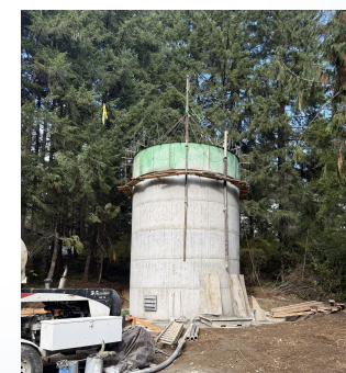
The reservoir being constructed
