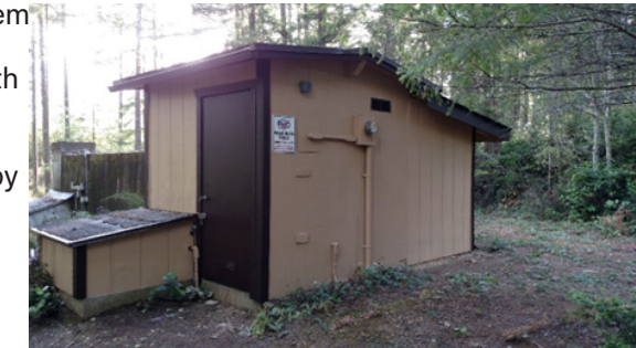
Well and Pump House
